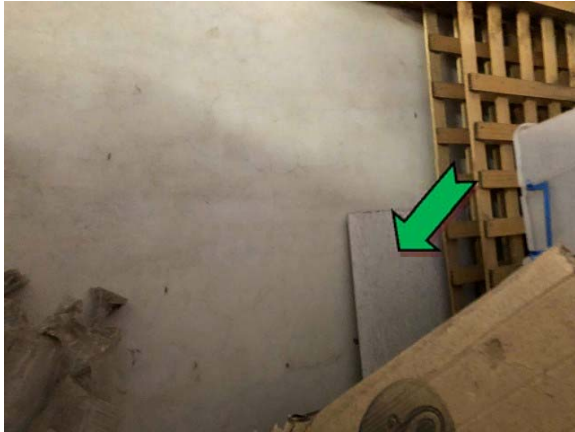
Photo 1. Interior, north elevation, store room, stored material – non asbestos-containing fibre cement sheeting.
